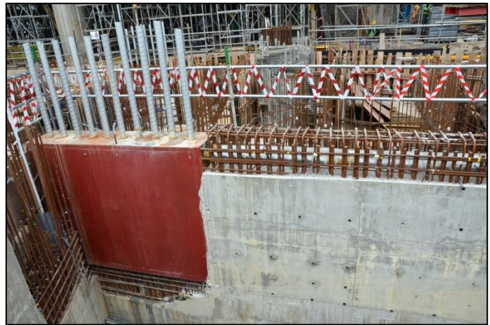
Special steel boxes to contain the very high bursting forces of closely spaced vertical tendons
