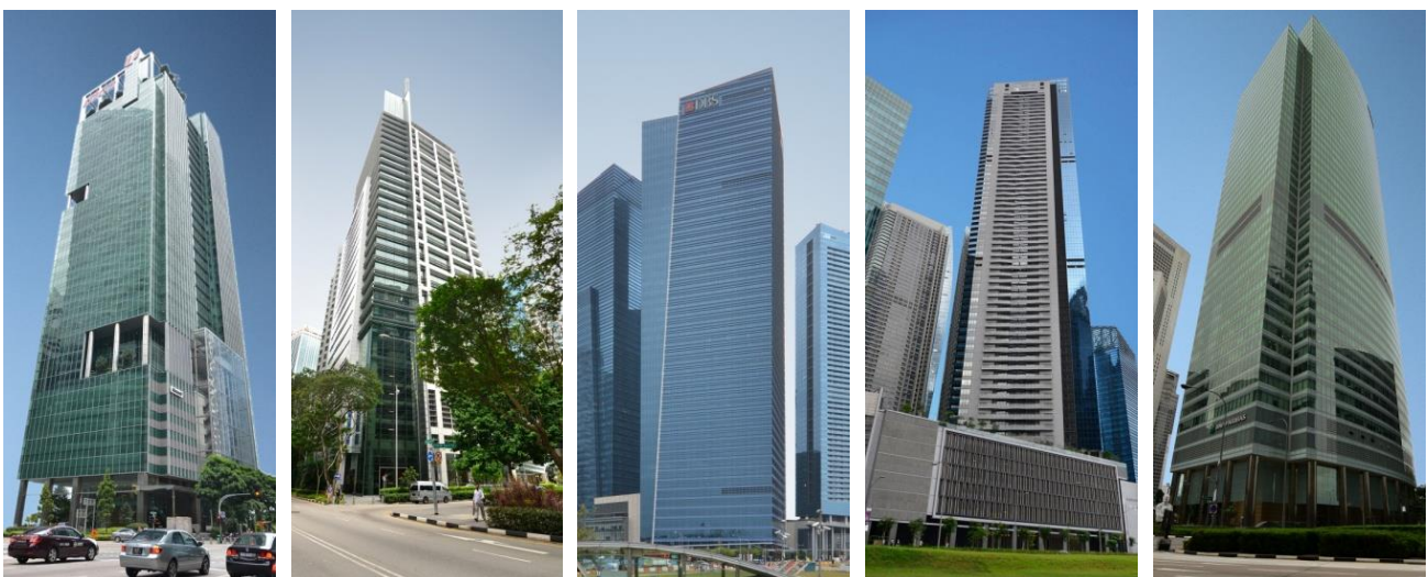
Post-tensioned high rise buildings in Singapore
