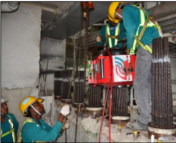
Stressing of vertical tendons in progress
