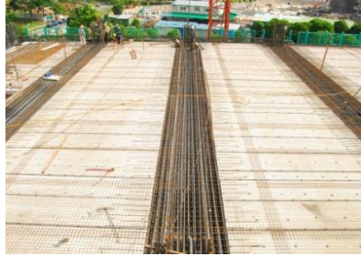
PT beam with PC slab
