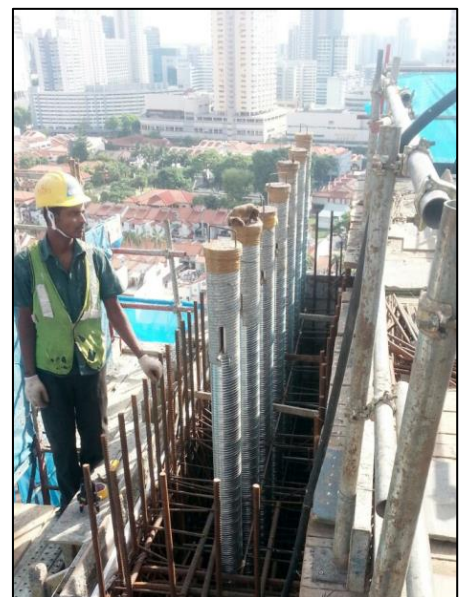
Installation of vertical tendons' ducts prior to concreting
