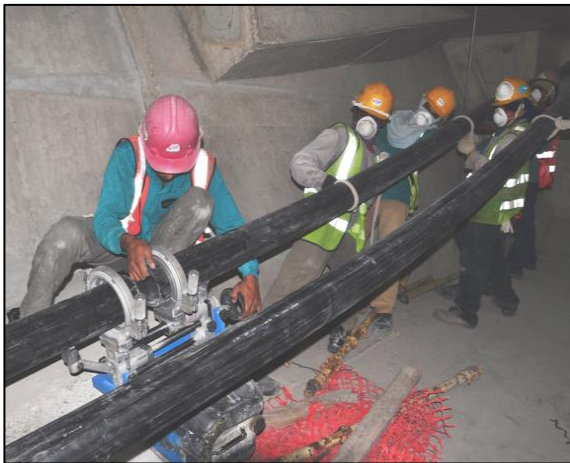
Individual lengths of HDPE ducts are joined together by mirror welding technique.
